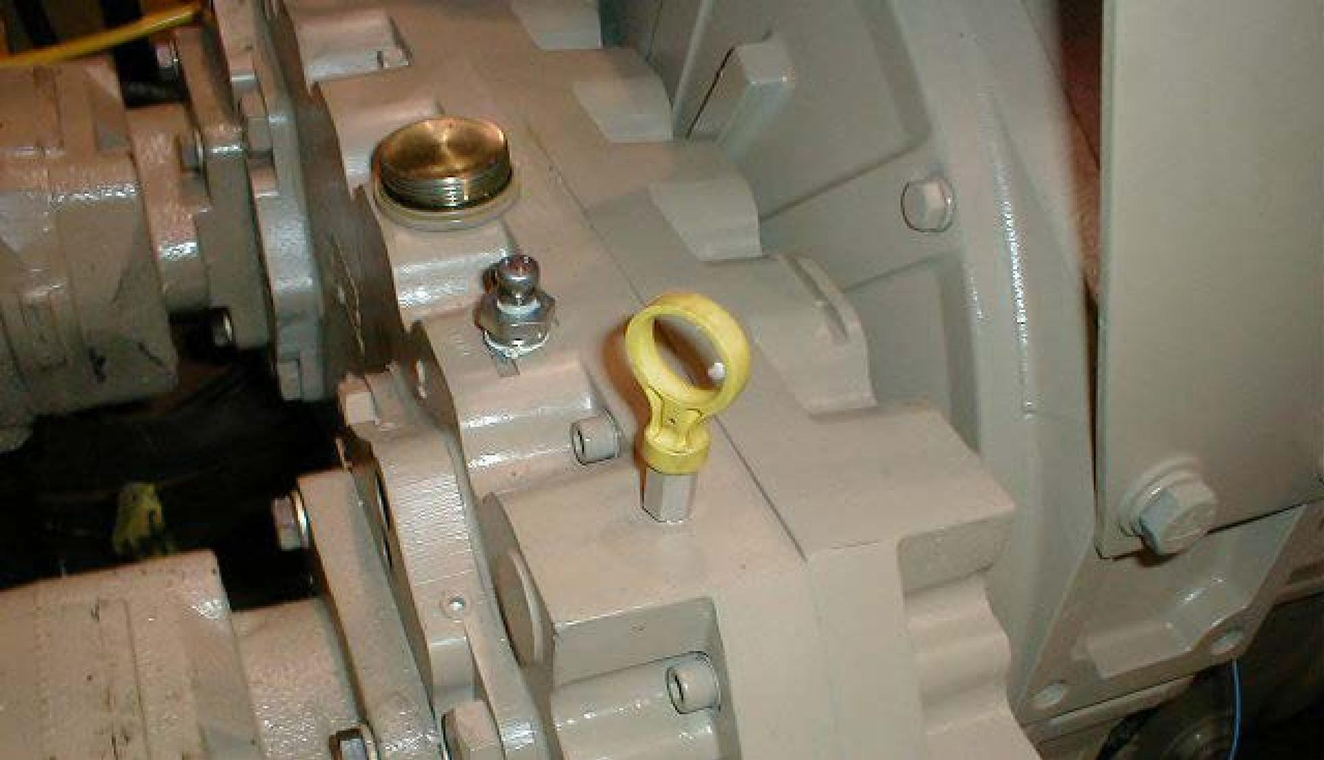
Check pump drive gear box oil level
